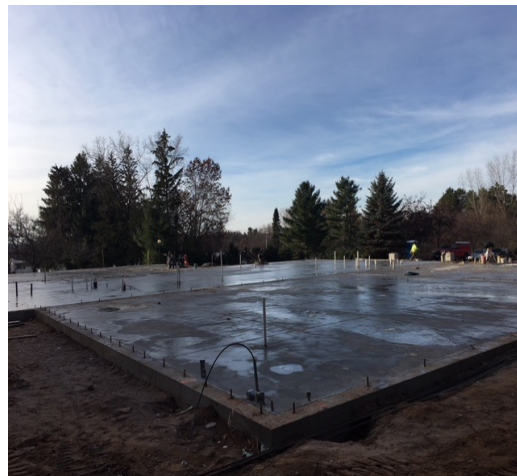
The entire slab is now finished! (Soon we'll see walls!)
